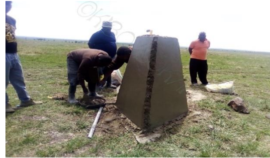
The reaffirmation and construction of 2 nd of 3 control points along the Kenya Tanzania international boundary at Nyabikongori Primary School in Migori County and at the Mara Traingle respectively.
